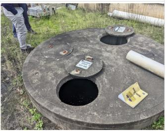
Plate 4.16 Oily water separator for compressors
